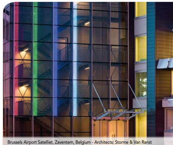
Brussels Airport Satelliet, Zaventem, Belgium - Architects: Storme & Van Ranst
